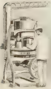
FILLING BY MACHINERY
